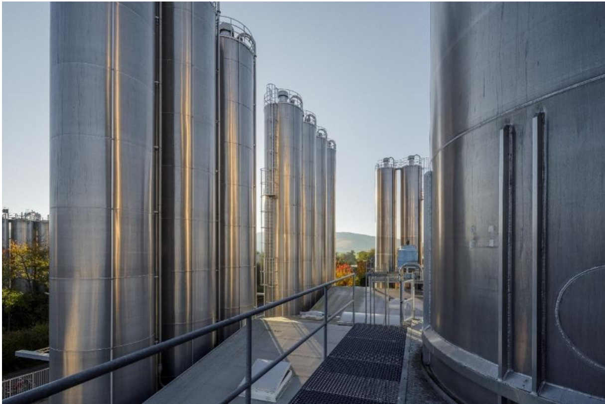
Photo of plastic silos belonging to Polyblend GmbH at the Bad Sobernheim site.
